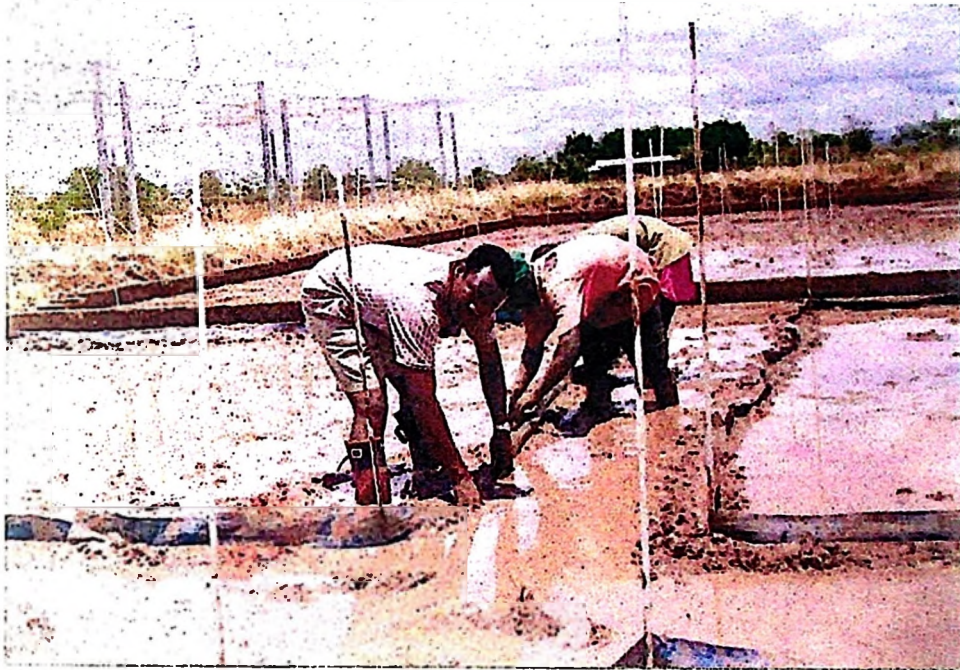
(a) Installation of impervious polythene sheeting in the plot boundaries
