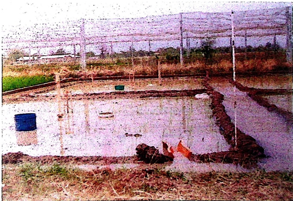
(b) Raising of earth bunds controlled irrigation
