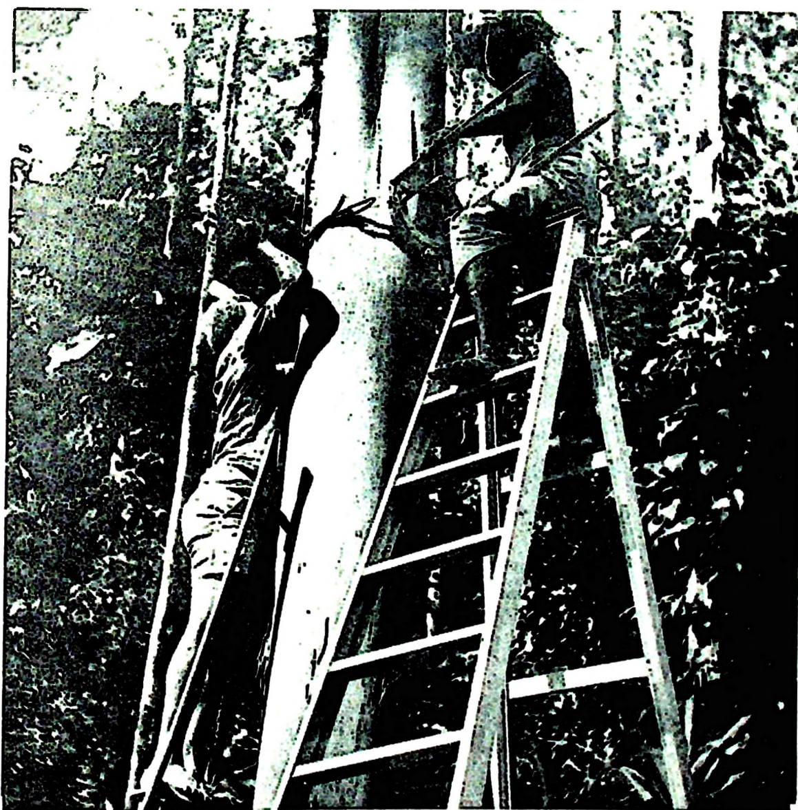
PLATE 12.4 Sampling for wood quality in standing trees of E. deglupta . The gimbal for the sampling machine (see Sulc, 1967) is being attached at a point 5 m above ground (10 per cent of total tree height).
