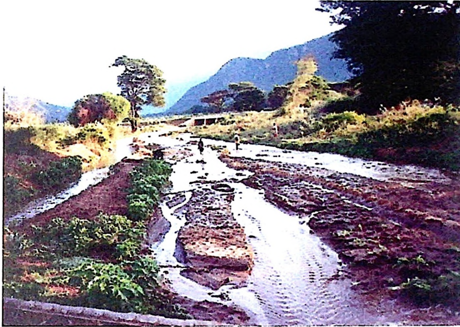
Plate 2: Runoff rainwater diverted into main field channels at Makanya Road Bridge
