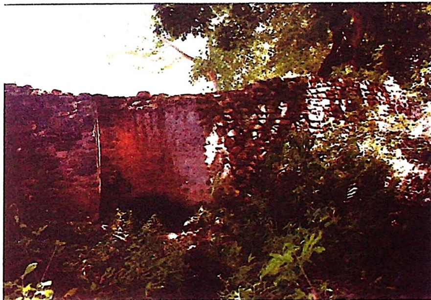
Plate 1: Micro-dam ( ndiva ) made of stones
