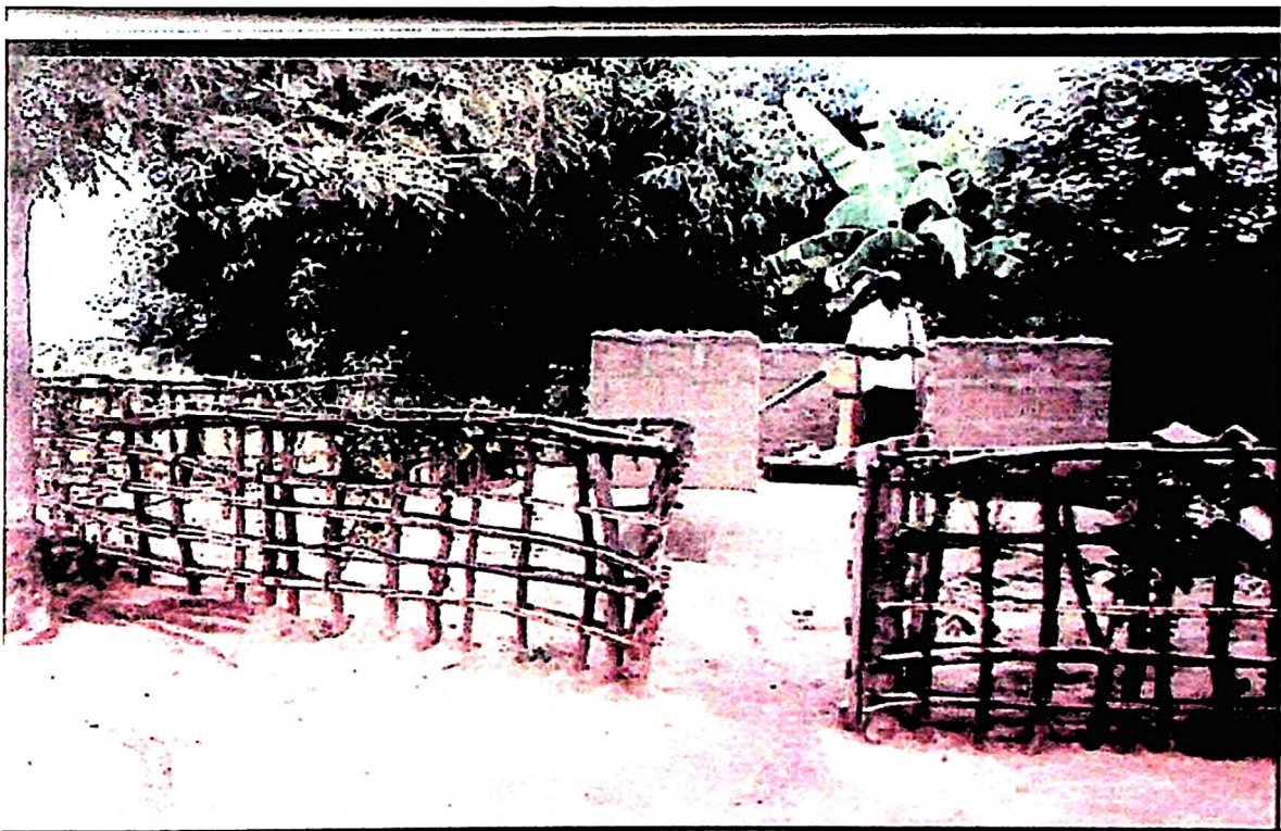
Figure 11: A deep well at Kahama village in Mwanza City.
