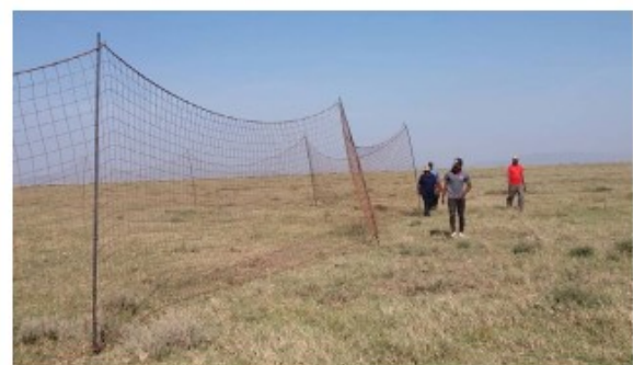
FIGURE 2 Picture showing netting structure with pipes inserted into ground pinned metal bars and hanging nets
