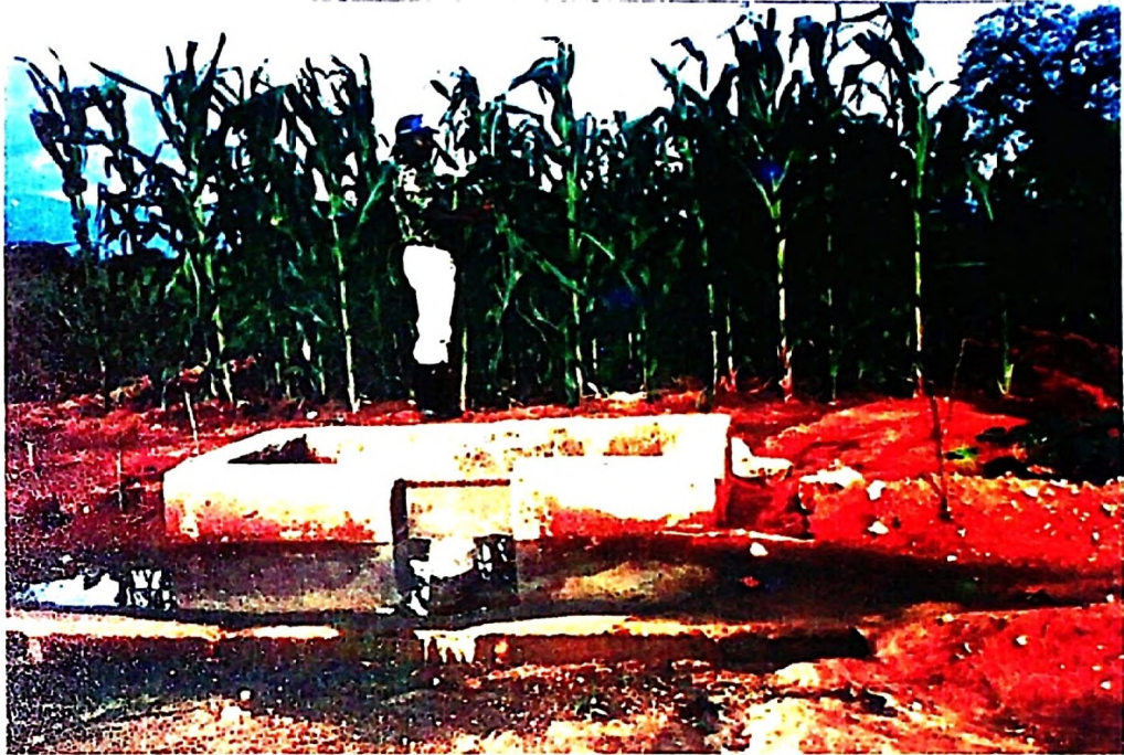
Plate 1: Storage tank with an apron and silt trap.
