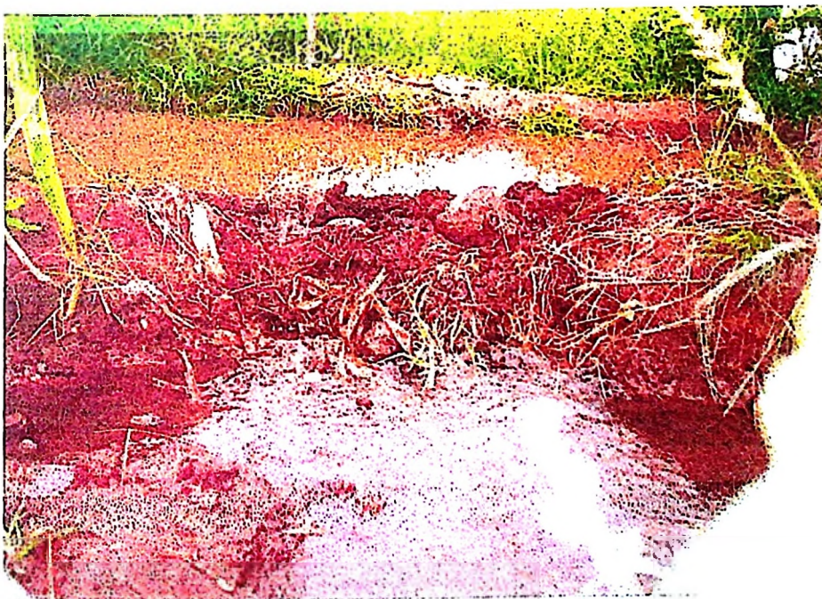
Plate 4.2 Distribution of water using grass and mud (earthen distribution box).
