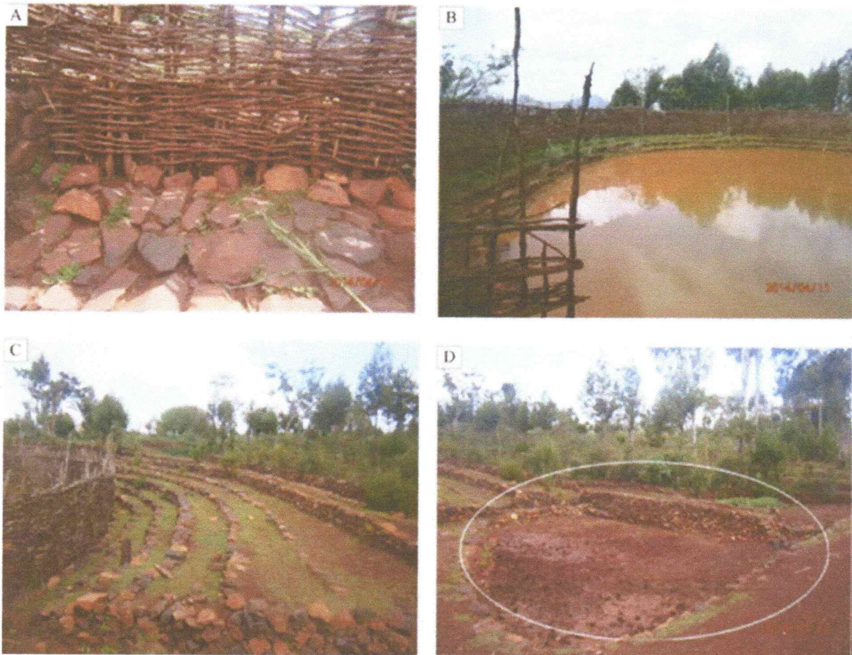
FIGURE 21.1 Water harvesting structures of the Konso people of Ethiopia. (A) A wooden mesh to filter out debris in runoff from entering the pond, (B) a fenced pond, (C) terracing outside to prevent silt from entering the pond, and (D) a stilling basin that settles silt in runoff before entering the pond. Adopted from Behaihu et al. (2016) .
