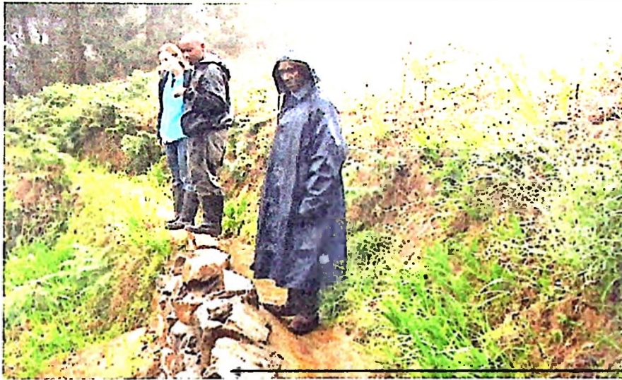
Figure 11: A repaired portion of broken Fuku canal
