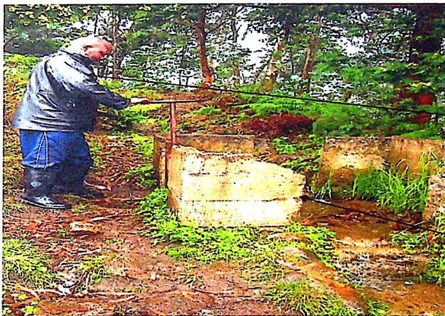
Figure 10: A broken division box of Fuku canal
