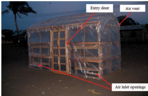
Plate 1a: The general structure of the solar tent (Front view)
