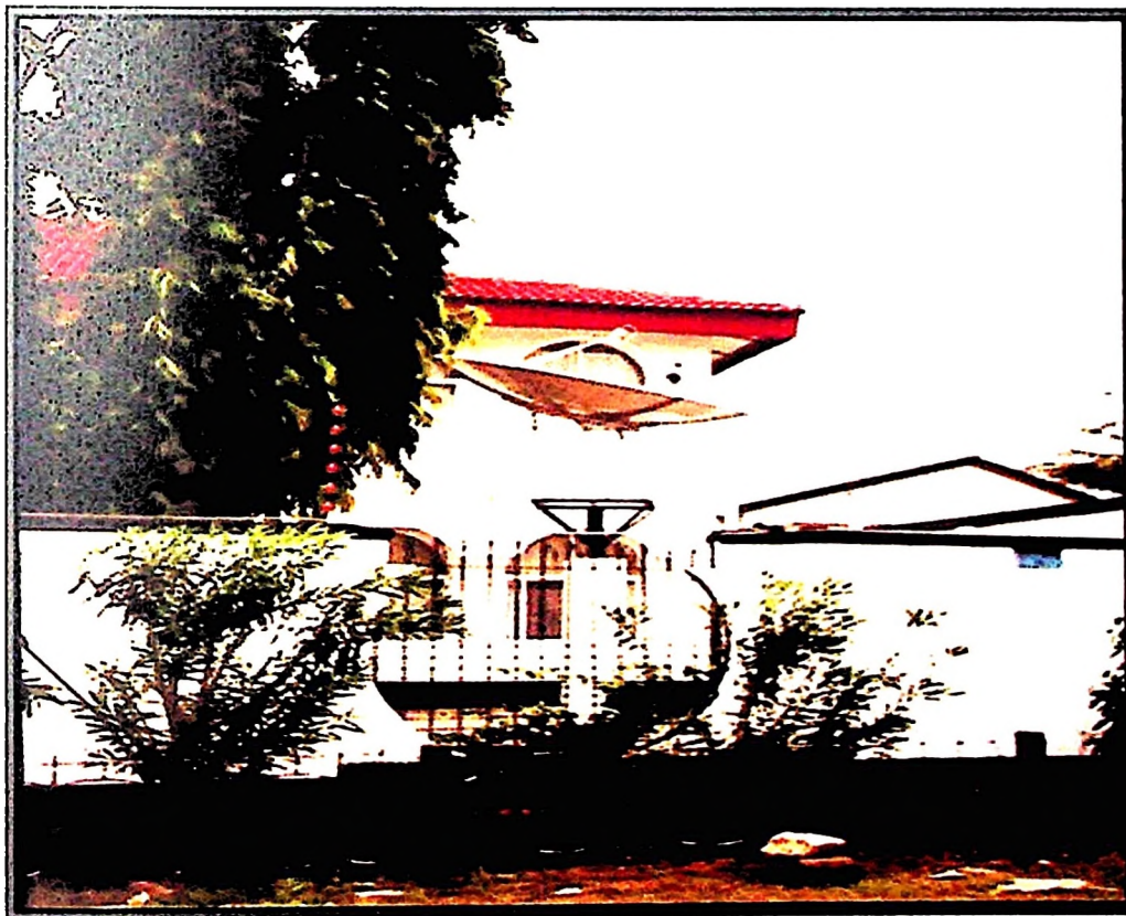
Figure 6: Effects of planting Polyalthia longifolia (Ashoki) on TANESCO power lines at Msasani area.
