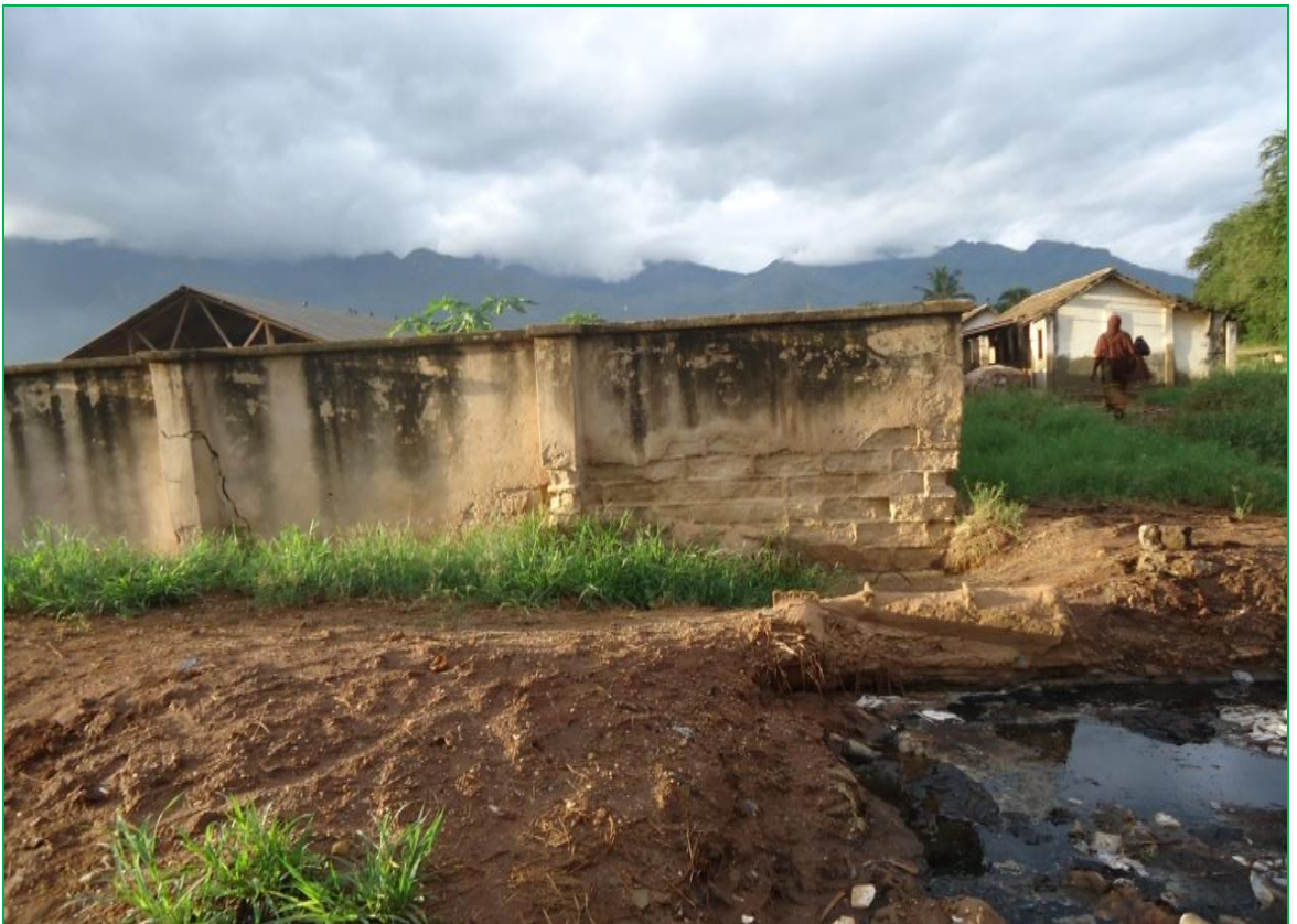
Figure 4: Abattoir walls with cracks and well containing water
