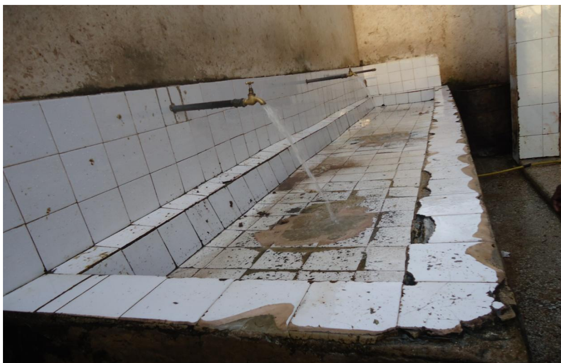
Figure 9: Wearing of trough with broken water tape
