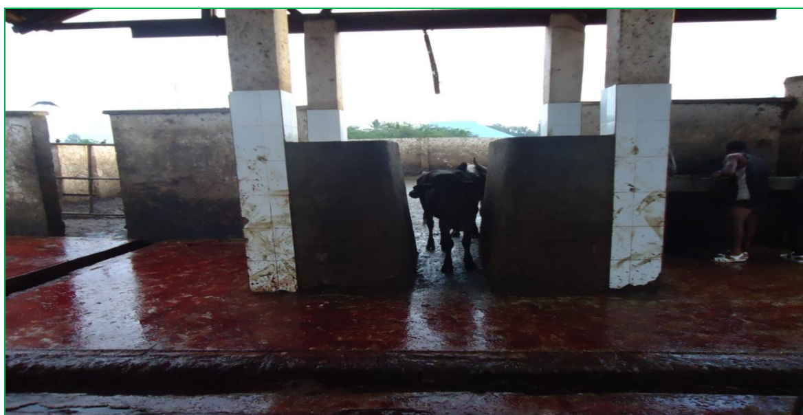
Figure 7: A poor hygienic condition of killing area and drainage canal
