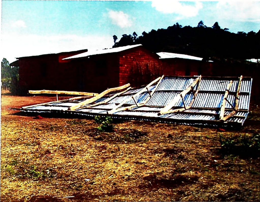
Plate 7: A house roof removed by unprecedented strong winds in Makonga village in the year 2007
