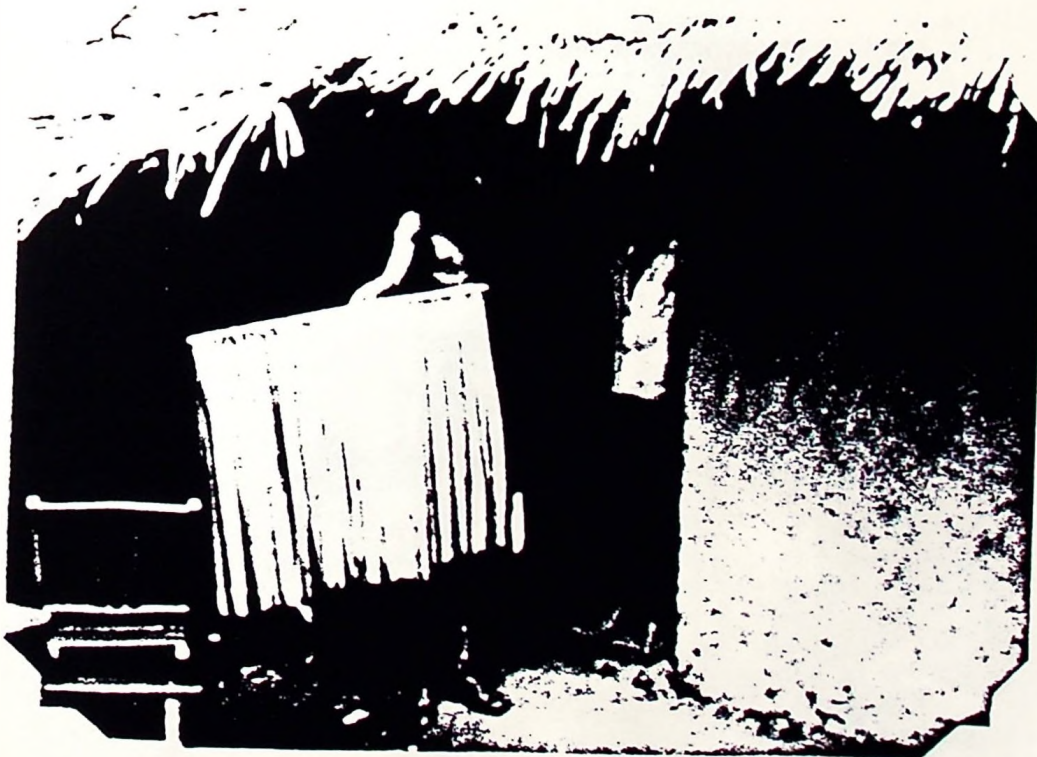
6. Coconut Palm Roofing Used for the Temporal Type of Housing
