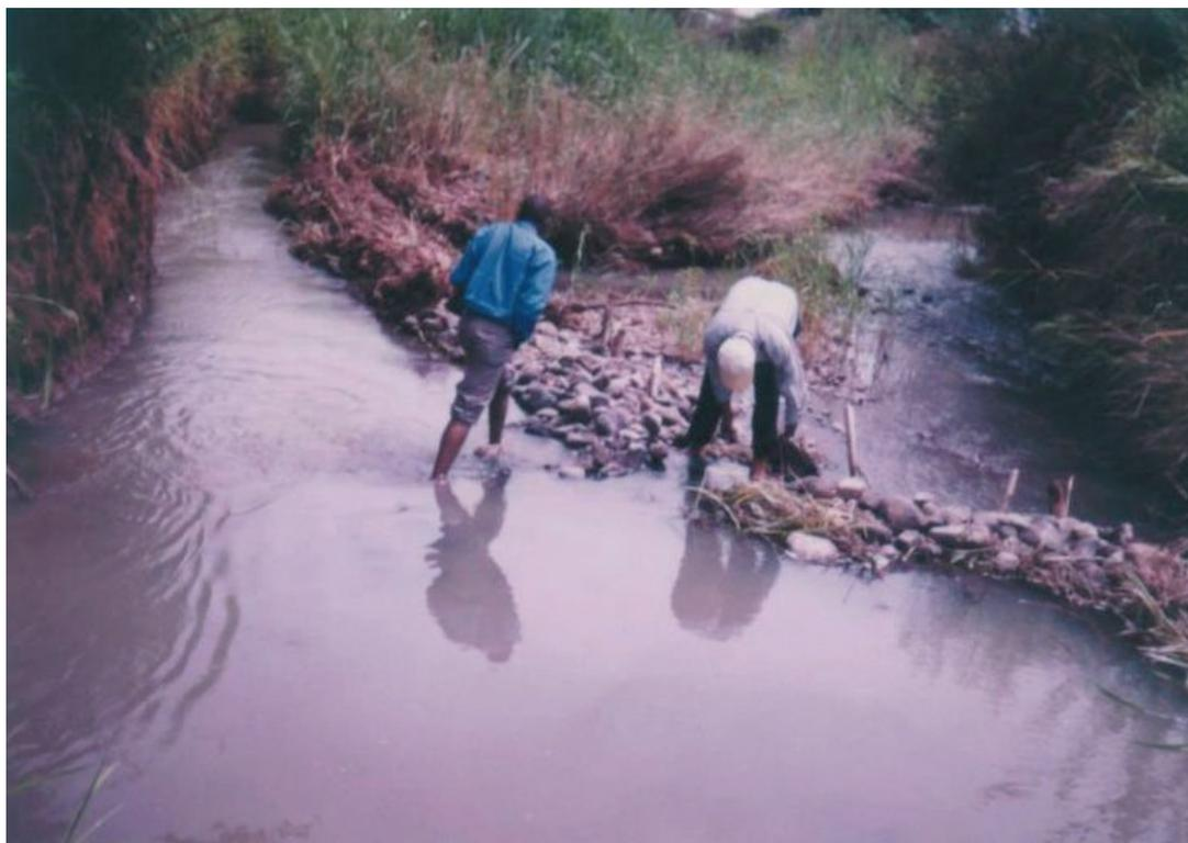
**Plate 1: Intake of Kalanzi Traditional Irrigation Scheme.**
