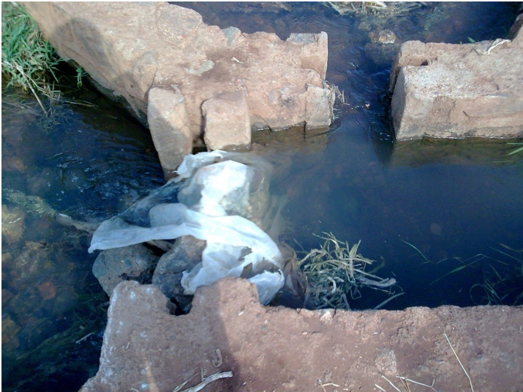
Figure : A division box without a stop-log
