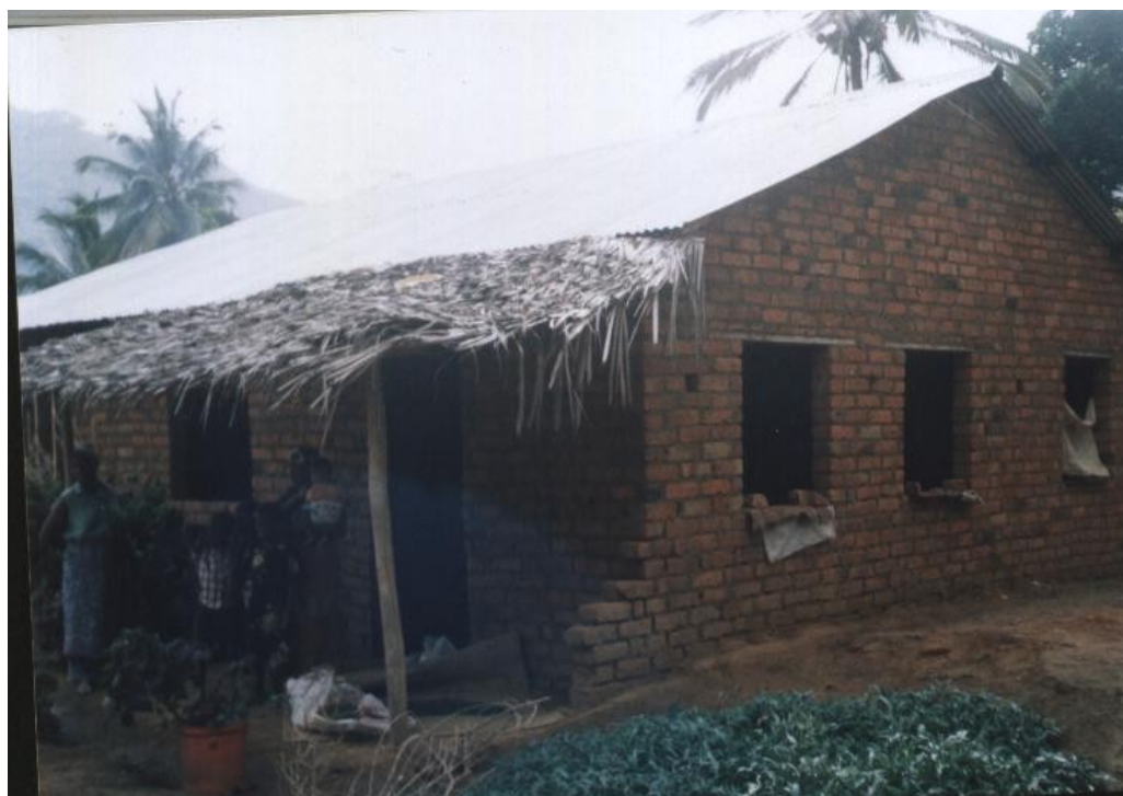
Plate 1: A newly constructed brick house at Chemka in Shebomeza village, around ANR, Tanzania
