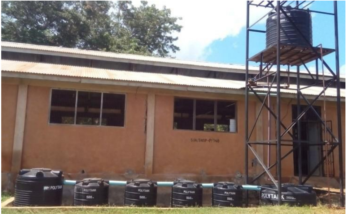
Plate 2: The water treatment system of the fish hatchery building at Aquaculture Research Facility- SUA
