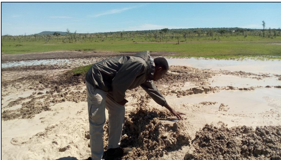
Plate 2: Water point damaged by elephants in Makundusi village, western Serengeti
