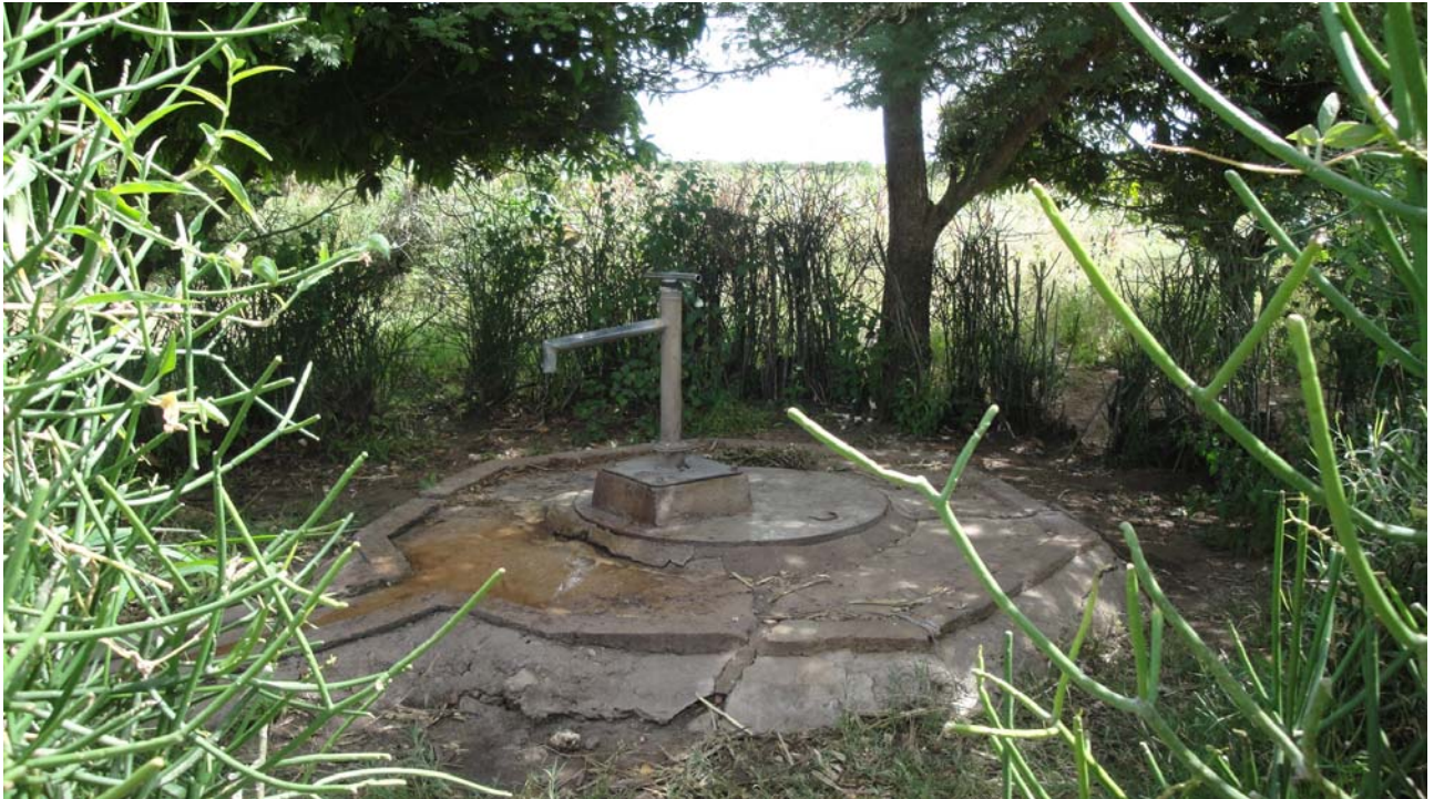
Plate 5. A non-functional water pump due to sub standard concrete
