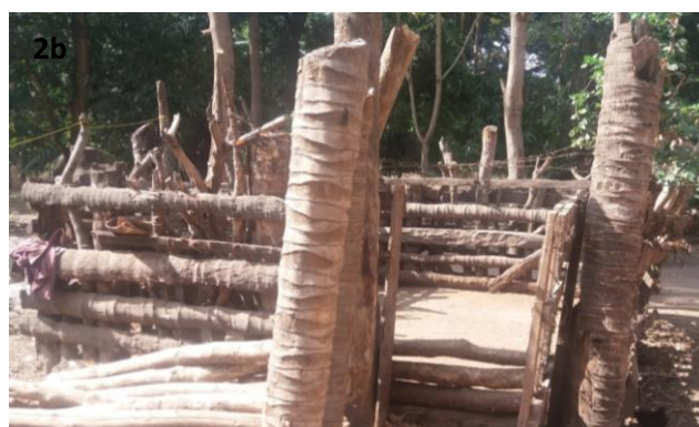
Type 2b. Open roof wood Boma: Ilonga
