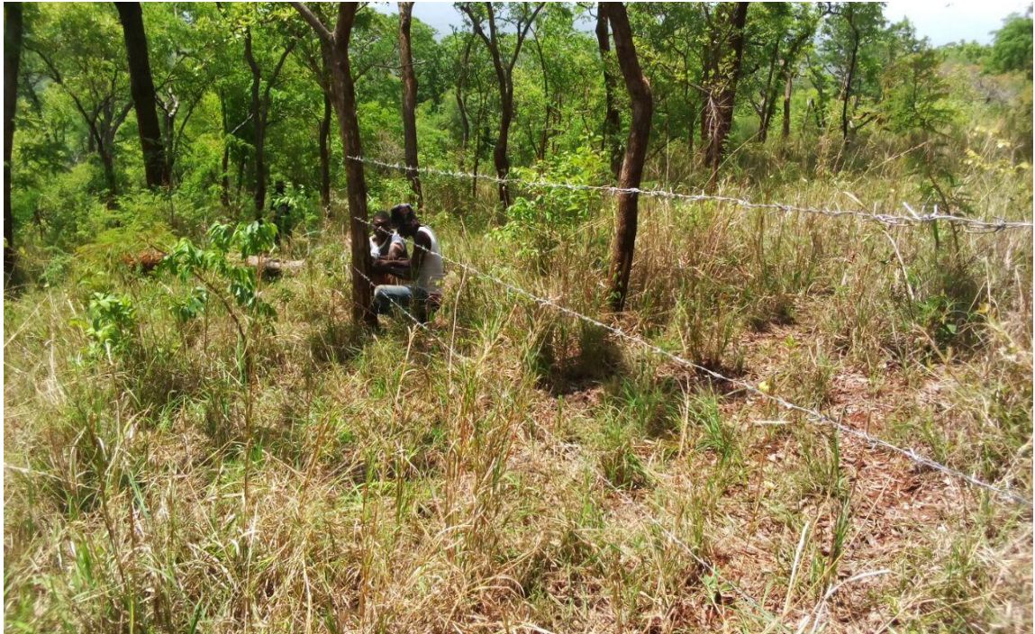
Plate 2: Photo showing wire fence construction of grazing plot in Ihombwe village, Kilosa, Tanzania: Source by researcher (2017)
