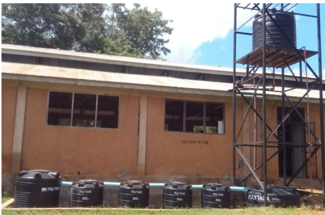
Plate 8: The water treatment system of the fish hatchery building at Magadu farm
