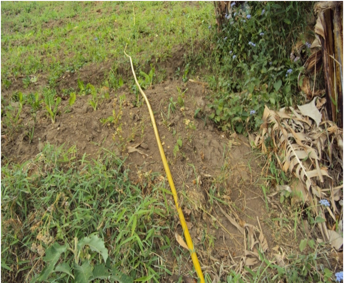
Plate 2: Water pipe lay on the ground flowing water from source to the field
