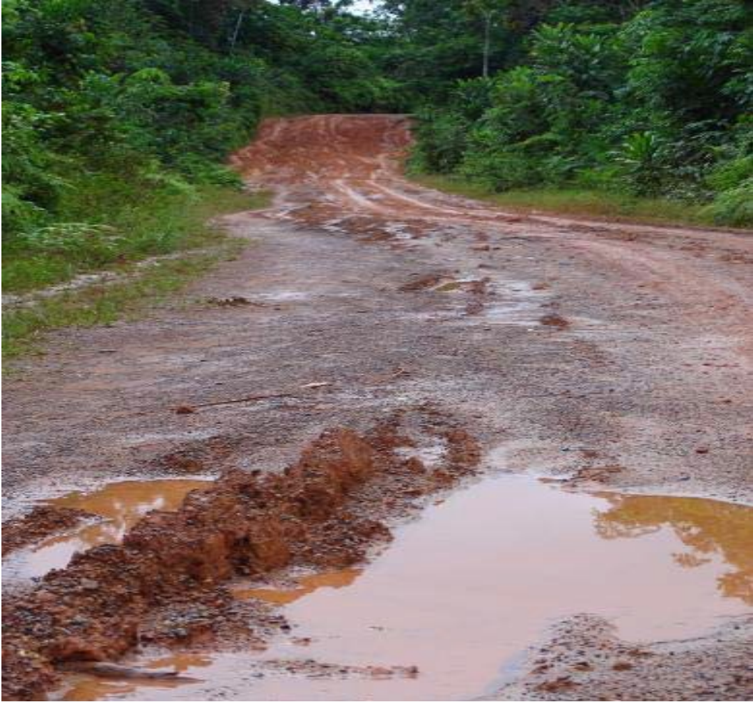
Plate 1: A road in sawala village
