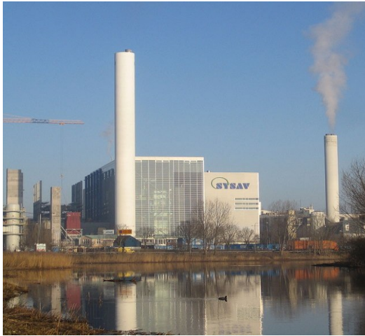
Plate 6: Incinerator in Malmö, Sweden
