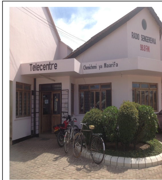
Plate 1.1: “ Sengerema Multi-purpose Community Telecentre (SMCT) alongside with Community Radio ” in Sengerema District, The biggest public owned telecentre in Tanzania. (ELEV: 3914ft S02 0 38.998' E032 0 38.627')
