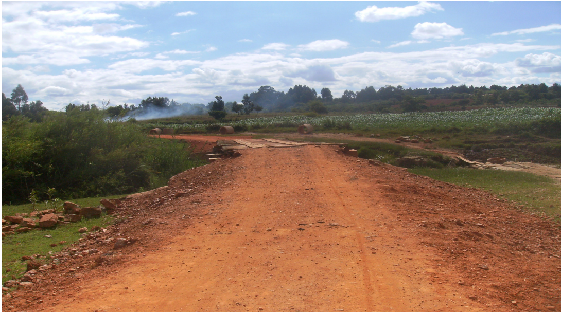
Figure 4: One of the bridges constructed by VTTP in Ukumbi ward
