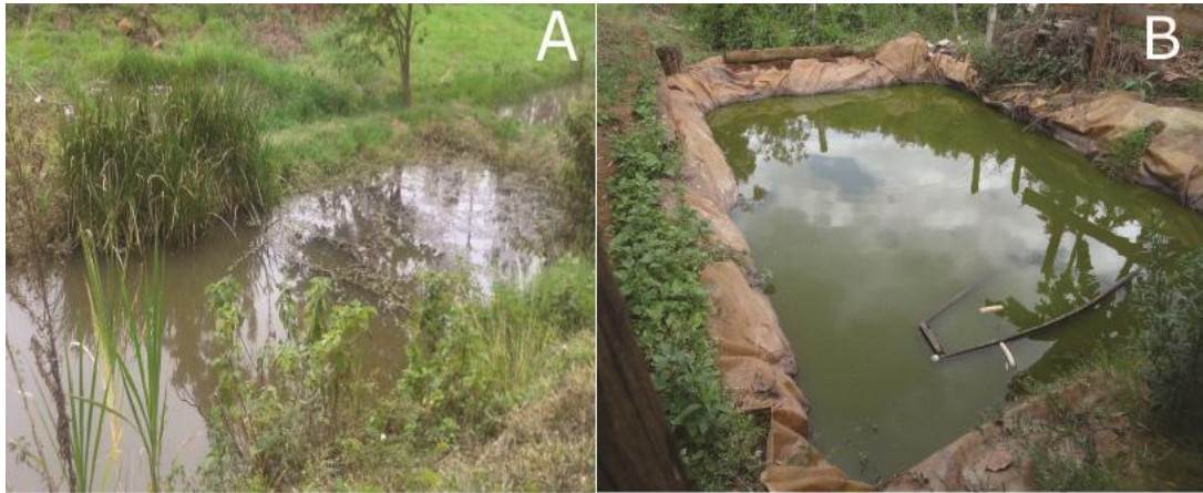
Figure 7: An earthen pond (A) with overgrown vegetation and a poorly managed liner pond (B) with collapsing walls and litter in it
